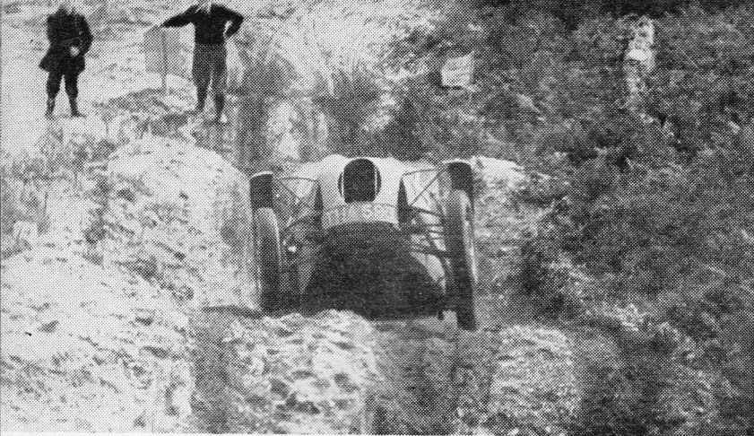
★ TOE-IN: (Left) Something more than the usual one-eighth of an inch is taken on by the front wheels of Deeley's Cran- ford at "Big Dipper".
