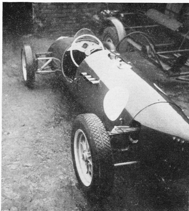
NEW contender for Formula 1 honours is the Gleed, which takes advantage of the 750 c.c. (S) section of the formula. Chassis is a lengthened early-type Cooper 500 c.c. model (left).
