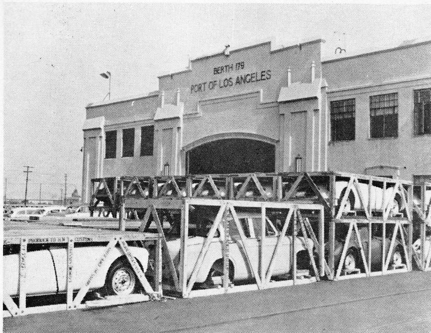
*BRITISH CARS for American drivers. This impressive display of crated cars include M.G.As and Hillman Minxes. The crates are open-sided and collapsible which simplifies shipping enormously.*
