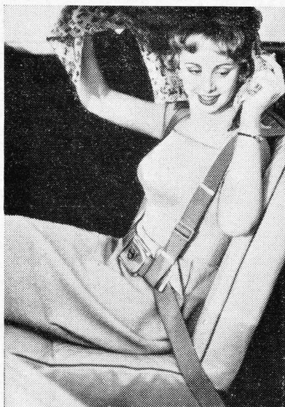
(Above) The Masco-G safety belt and harness conforms to British Safety Council standards. It incorporates an adjustable quick-release buckle.
