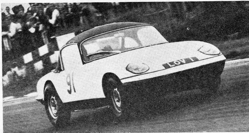
camber of the front wheels has been very carefully set and the rear wishbones are of the latest Lotus type which are adjustable for toe-in.
