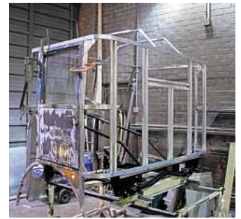
ABOVE: The cab had to be completely rebuilt. PHOTO JOHN SULLIVAN.
