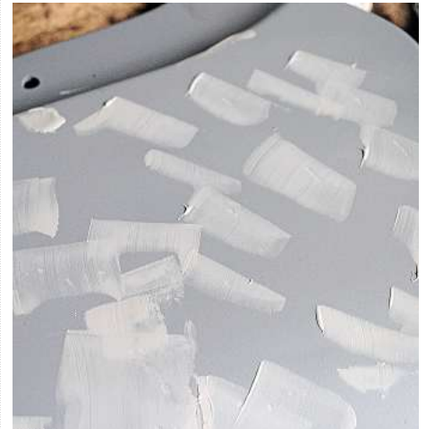
14 Acrylic or stopping putty is an extremely thin filler, it needs to be applied in thin layers and allowed to dry thoroughly before sanding down and repainting; if rushed it will inevitably "sink" leaving blemishes in the finished paint work.
