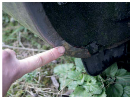
Rust tends to start on the arches.
