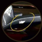
Mirror Arm Corrosion
